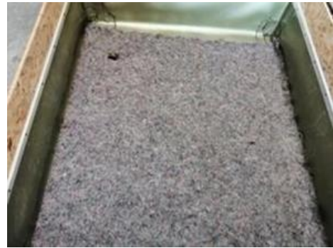
Figure 4 Second geotextile felt moisture trap placed on ecb geomembrane
