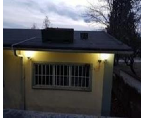
Figure 11 Green roof system, solar energy system and garden lighting
