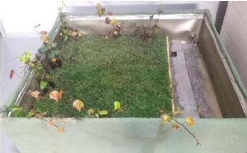
Figure 8 Extensive green roof
