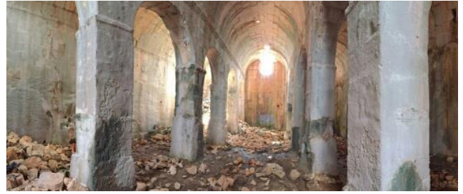
Figure 3. Interior view of Akkale Cistern
