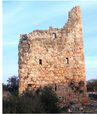
Figure 7. Hellenistic period Tower constructed with polygonal masonry technique in Kanlıdivane
