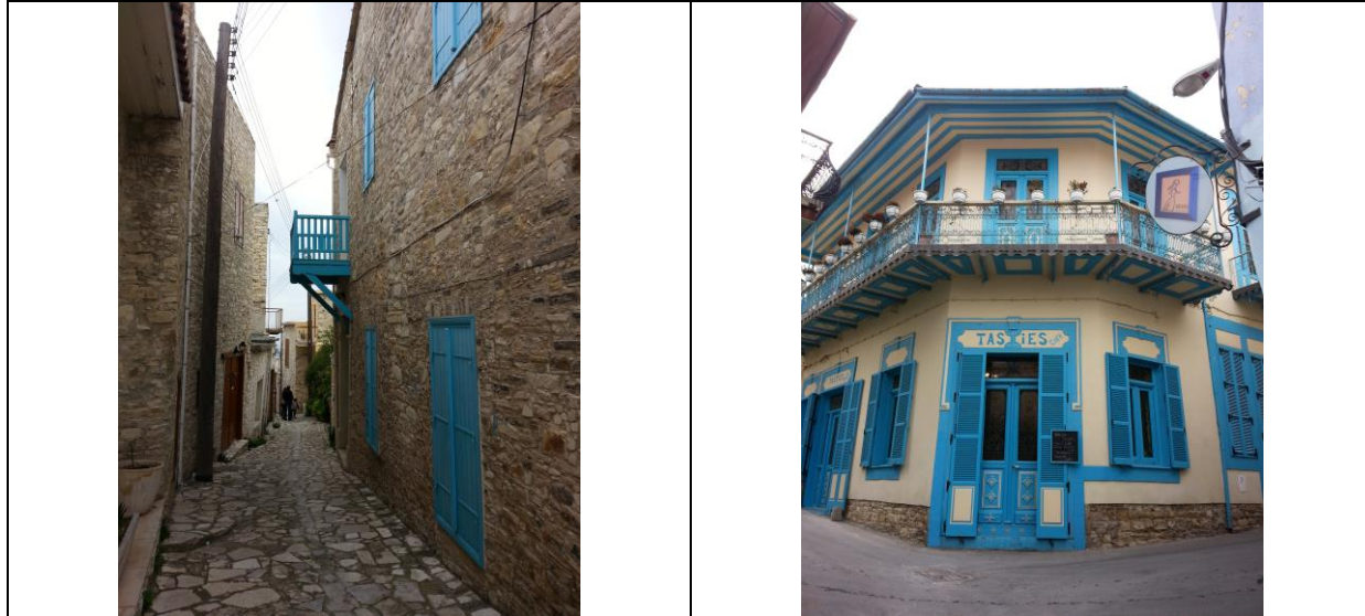
Figure 5. Change of façade and architectural elements. (Photo: Author, 2019)
