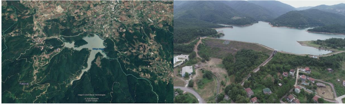
Figure 2. General view of the reservoir area and body of Gökçe Dam (Damla, 2020)
