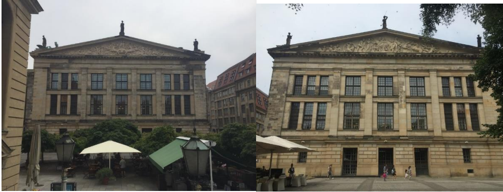
Image 19: The north and south facades of the Schauspielhaus.
