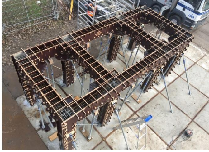
Figure 5. CAST Formwork System (CAST Formwork System, 2017)
