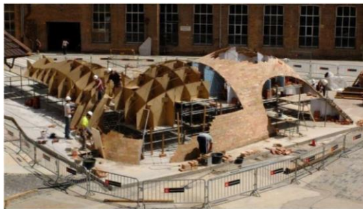
Figure 10. Construction process of the Catalan vault [37]
