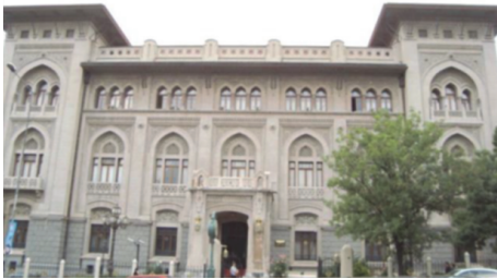
The Ziraat Bank Headquarters building in Ankara
