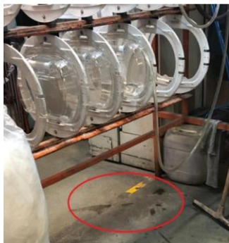
Figure 9. Water spill under the manual leak testing area
