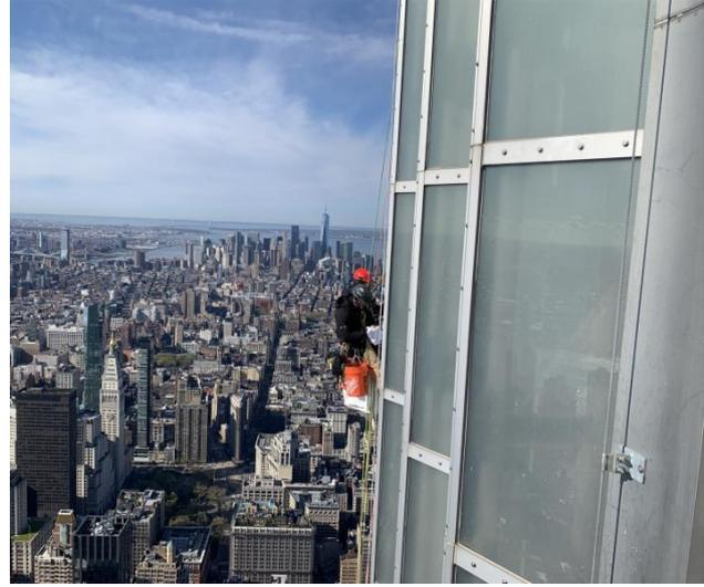
**Figure 2.** Maintenance work on the facade of the building (Mattani,2020)
