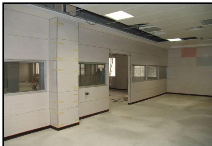
Şekil 6. Kompakt Laminant Duvar Görünüşü ve Mikrojaluzi Cam Panel Figure 6. (A wall built with a Compact Laminate covering and inserted a Micro jalousie Glass Panel)
