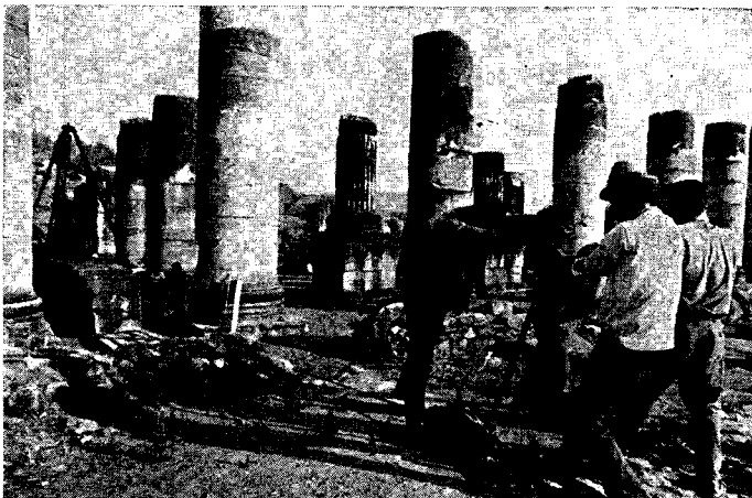
Fig. 19 — Artemis Temple : A 25-ton architrave block being moved to new position north of Church M.
