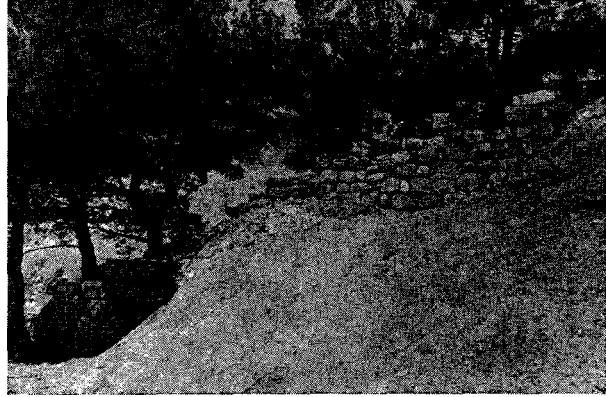
Fig. 24 — Pre-Hellenistic Defense Walls on the south side (AcS) of the Acropolis. At lower left, a triangular construction. Looking west.
