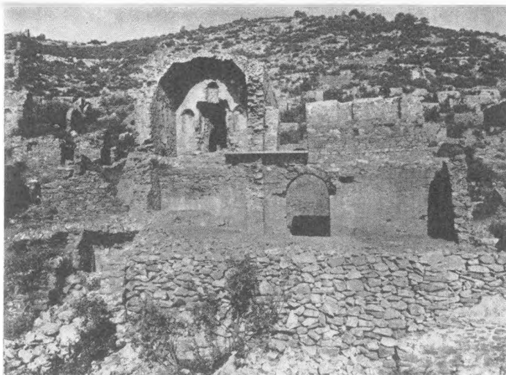
Fig. 6 — Anemurium, Tomb A II 14. East Side after Restoration.
