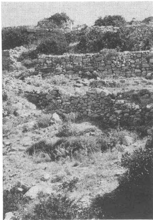
Fig. 4 Bottom of stepped street before excavation, showing modern terraces covering sections of street. Taken from south looking north.
