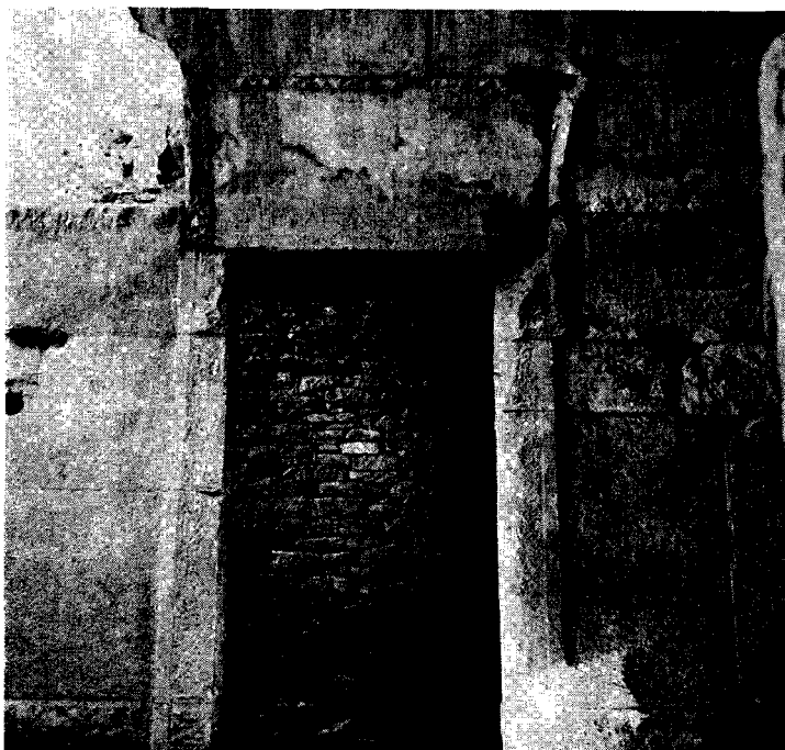
5 Theatre. Central vaulted tunnel of the stage building with door (cf. lintel inscription) communicating with side chamber,
