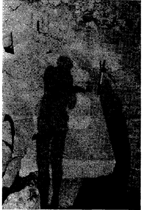
Fig. 14 — Byzantine Church D: outer wall of central apse made of curved, inscribed blocks, west to east
