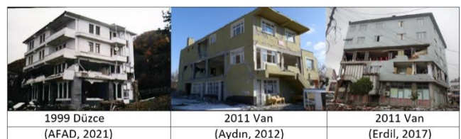
Figure 5. The substantial to heavy damaged (Grade 3) RC buildings
