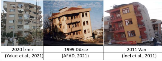
Figure 6. Very heavy damaged (Grade 4) RC buildings
