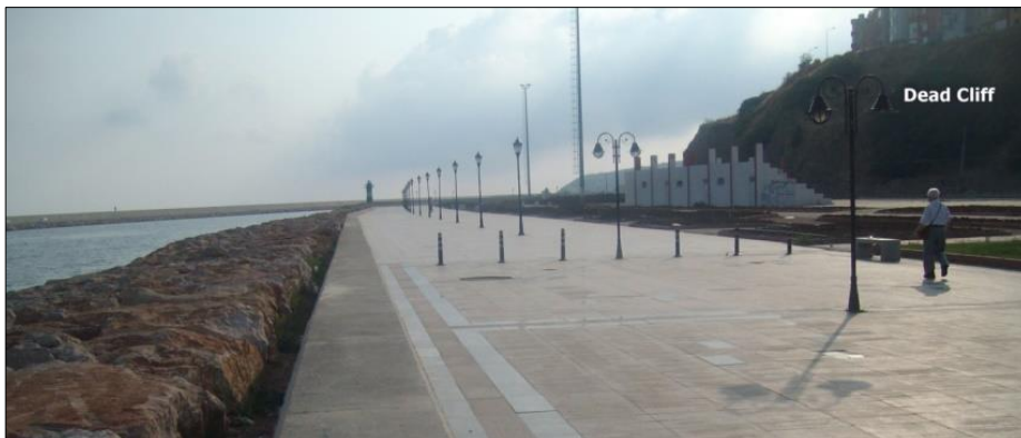
Photo 5: Coastal Landfills that Serve to the People of Bandırma as a Walking Area (2013).
