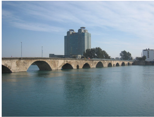
Fig. 2. Downstream Façade of the Taşköprü
