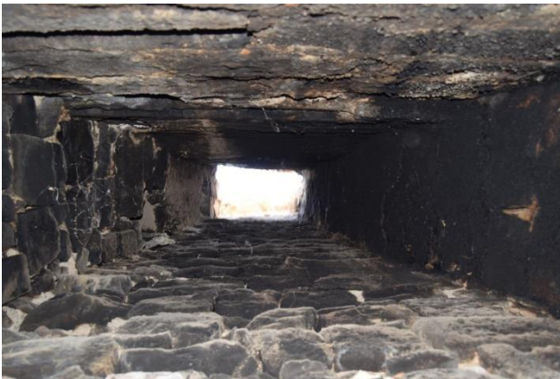
Figure 13. A view from inside the chimney
