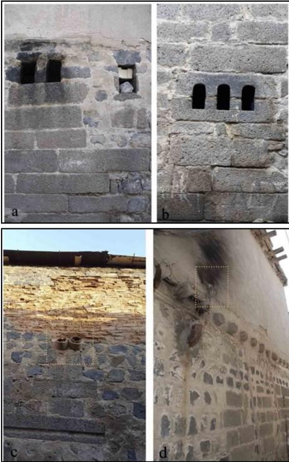
Figure 19. Examples of chimneys that evacuate smoke from the street facade
