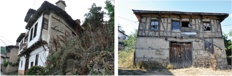
F. 7: Examples of traditional structures built with stone, soil and wood in Dağgüney and Süleymanbey villages (Güneş Kaya, 2019)
