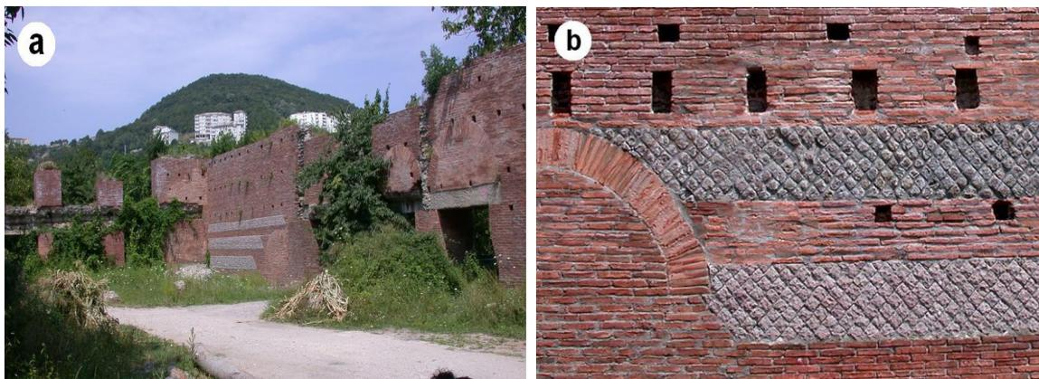
Fig. 2 [a] Basilica remains, [b] Opus reticulatum masonry
