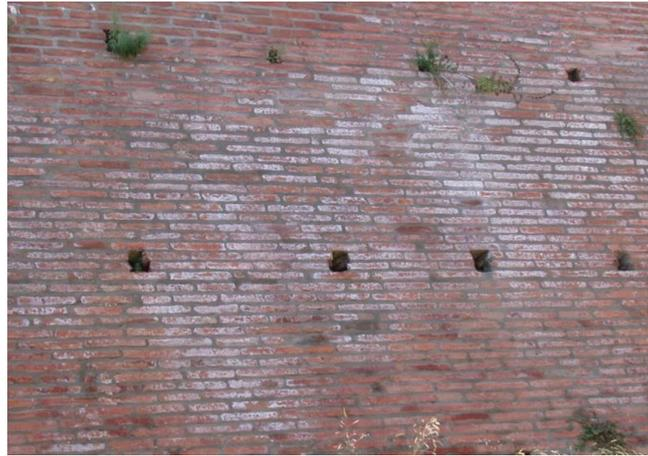
Fig. 3 Efflorescence on wall surface due to use of mortar containing portland cement binder during the previous restoration
