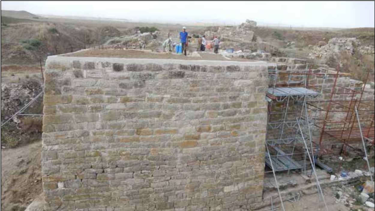
Fig. 6. East Citadel Gate: north face of the South Bastion following the installation of the soft-cap. (Photo by Brian Rose; courtesy Penn Museum, Gordion Project Archives.)
