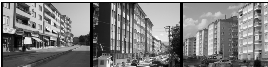
Figure 2: Typical Reinforced Concrete Apartment Buildings from Duzce, Cankiri, Corum
