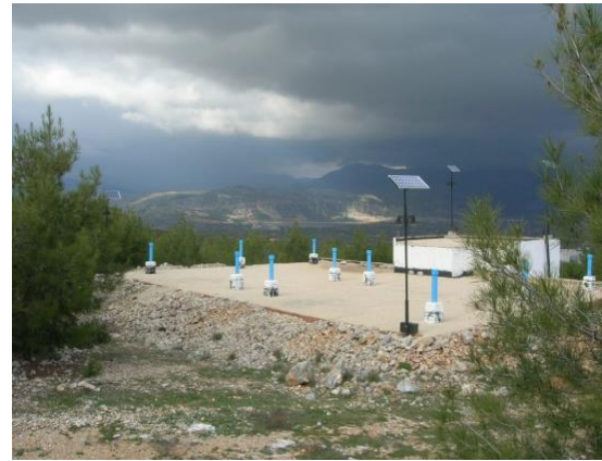
Figure 8. Lamp posts on the top of water depots.
