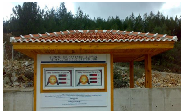
Figure 6. PV arrays on trackers and control room with displays.
