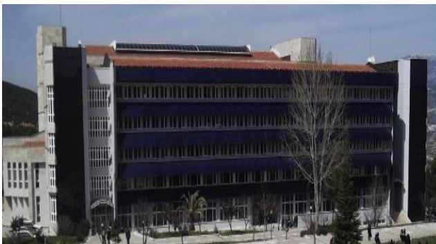
Figure 5. BIPV System on Façade.
