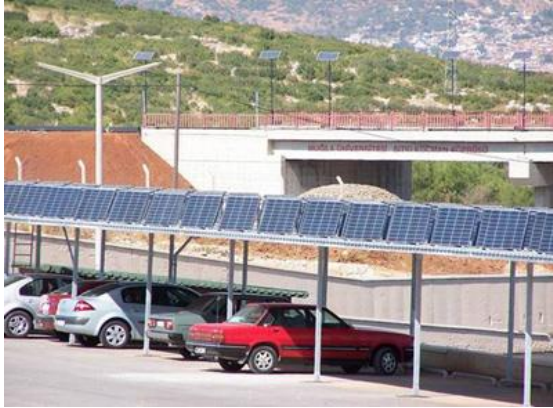
Figure 7. The hybrid car boot system (installed power is 15kWp) and lamp posts on Bridge.
