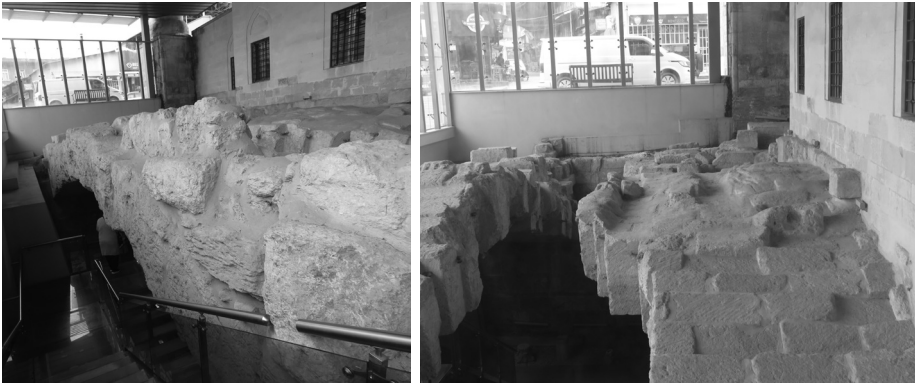
Fig. 2-3 General View of the Downstream Façade of the Bridge and the Top View of the Vault (Photo: İlkey Göçmen).
