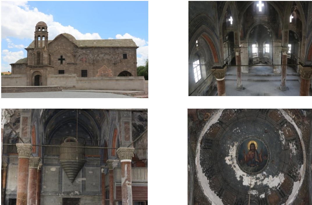
Fig. 1. a) Image of St. Theodoros Trion church, Nevşehir; b) view of apse; c) gallery floor; d) dome of St. Theodoros Trion church
