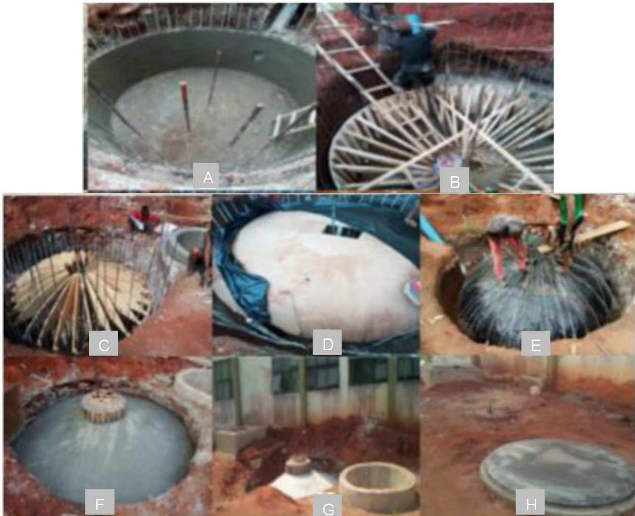
Fig. 2: Construction stages of the biogas digester plant
