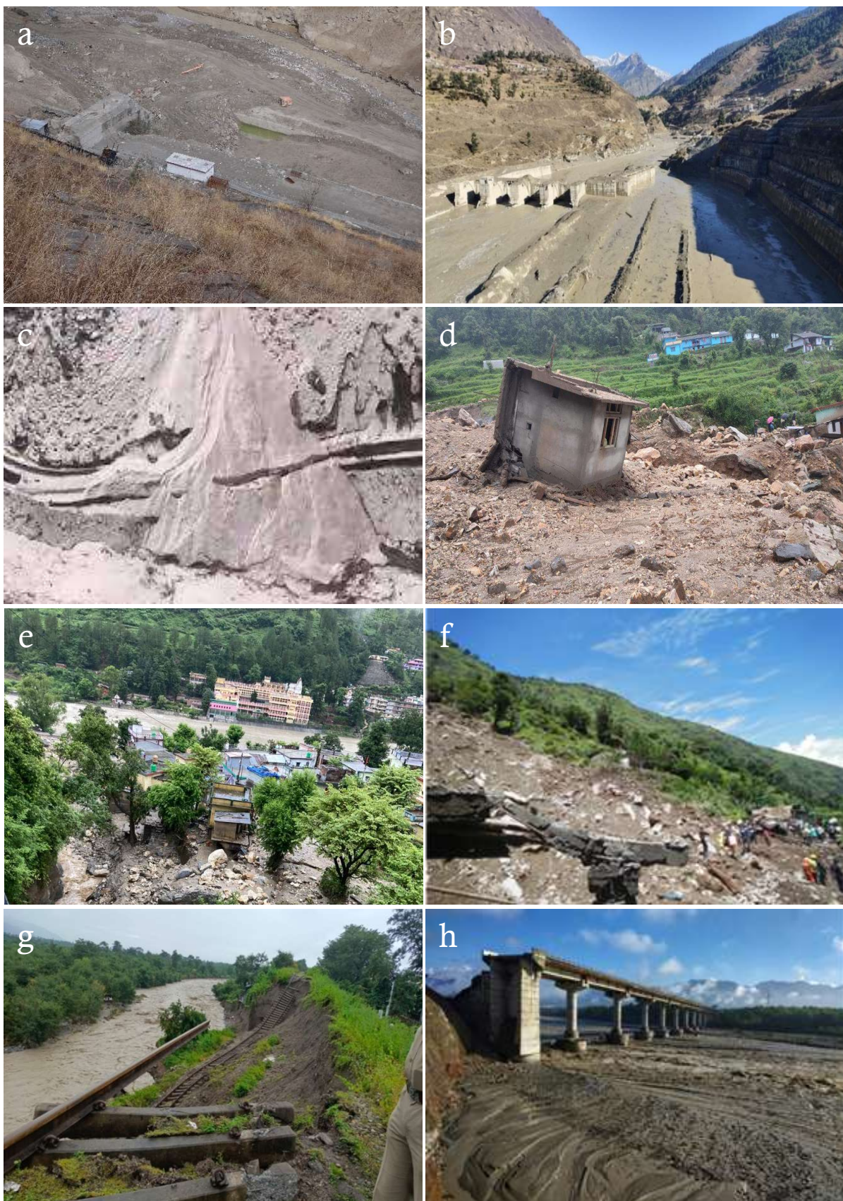
Fig. 4. Rock fall, flash flood/flood, avalanche and heavy localised rains or cloudbursts associated damages (a) washed away Rishiganga hydro project, (b) badly damaged Tapovan-Vishnugad hydro project, (c) an avalanche triggered near Sumna, (d) Ruined a house at Kankarari Village, (e) property damages in Mando Village, (f) damaged house at Jumma, (g) eroded railway track between Kathgodam and Haldwani and (h) damaged Gaula Bridge in Haldwani
