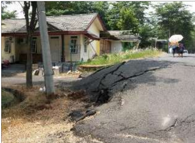
Fig. 1. Cases of civil structure damages induced by expansive soil
