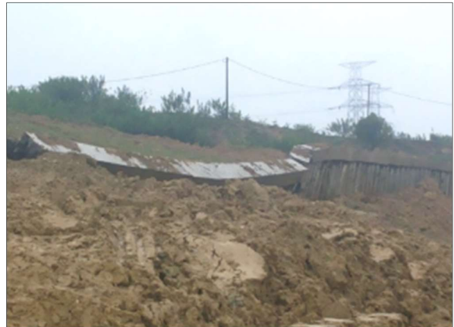
Fig. 1. Cases of civil structure damages induced by expansive soil
