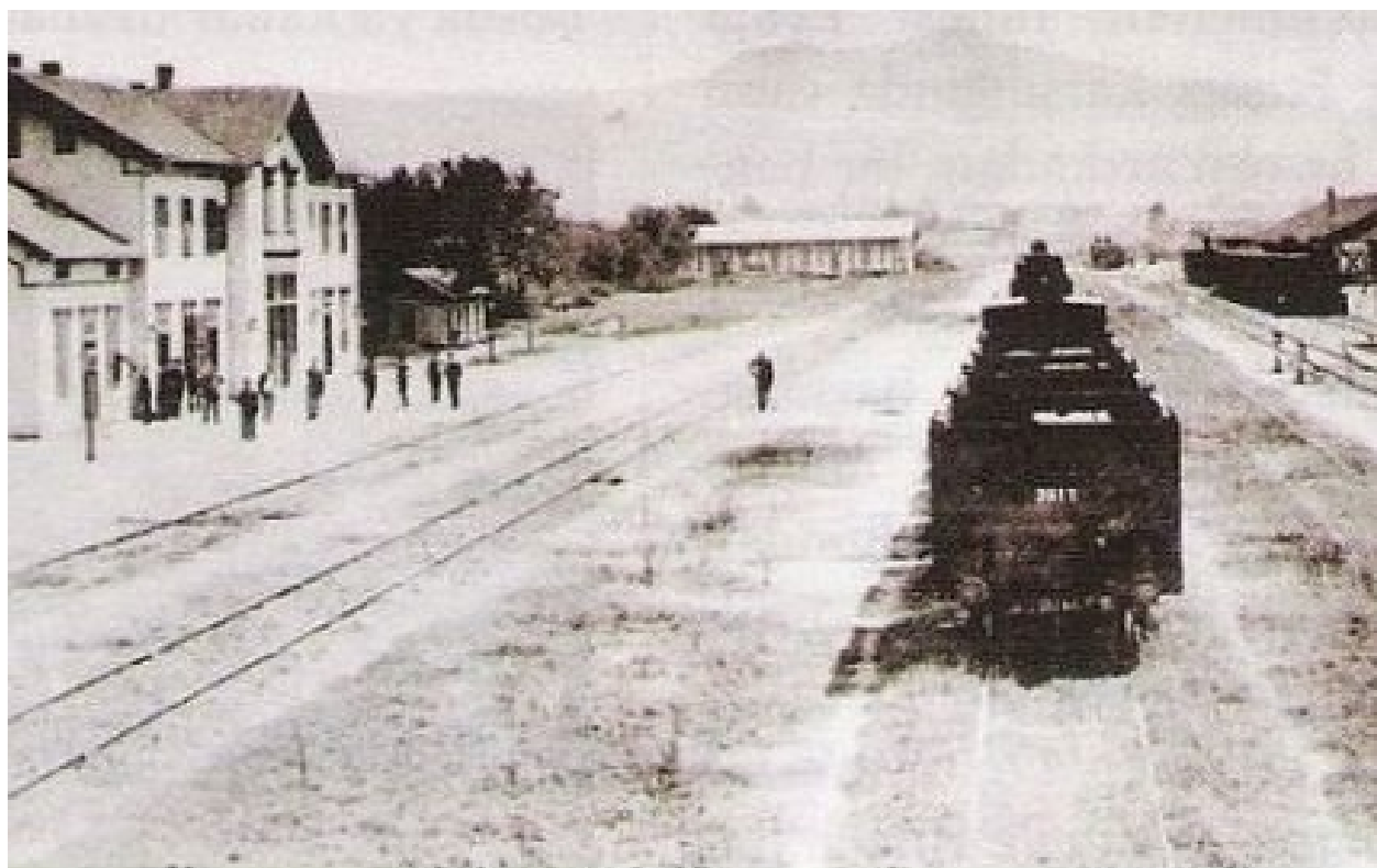
Figure 1: Rumeli Railway, Alexandroupoli Station
