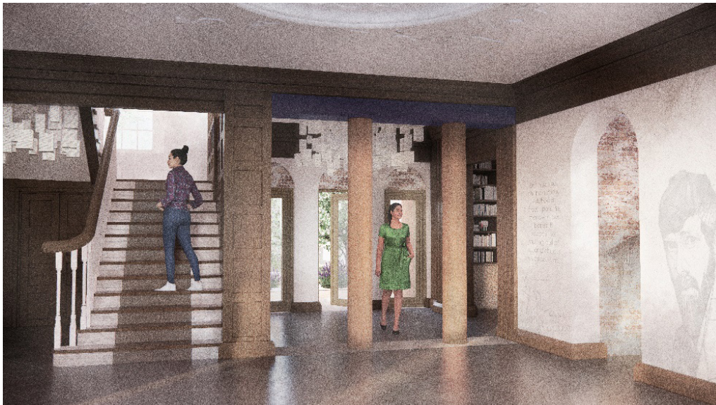
Figure 32. County House's original entrance chamber retains as much of the existing fabric as possible but balances this with the need to make repairs and to rationalize the internal layout. Floor tiles, where damaged, are swapped with travertine replacements formed using crushed brick from nearby demolition works, while traces remain of the timber Victorian staircase, removed and fitted elsewhere. New doors in the place of windows are picked out in brass, as are structural interventions.
