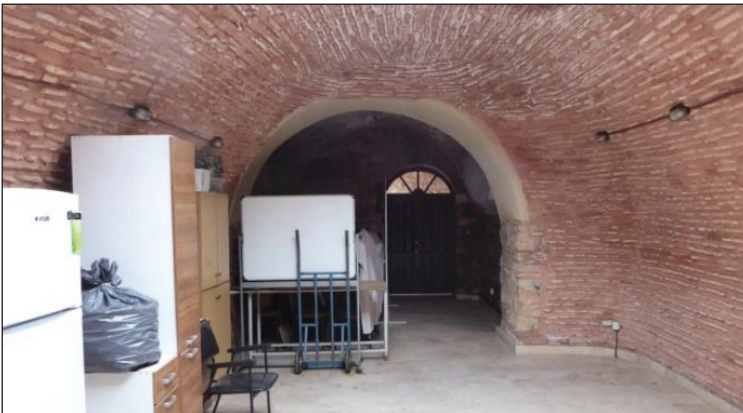
Photograph 11. It is the middle section inside the cistern.
