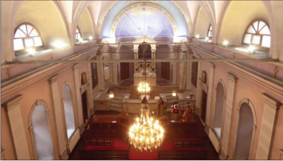
Photograph 5. This section is the naos section of the church.
