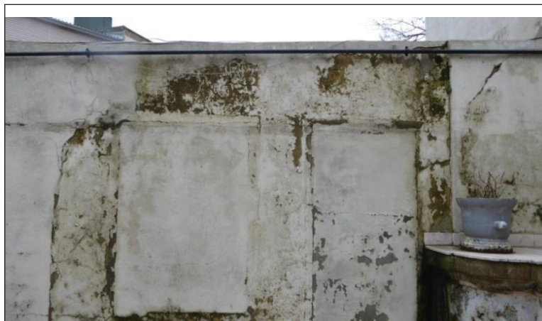
Photograph 28. The traces of the door can be followed on the wall.
