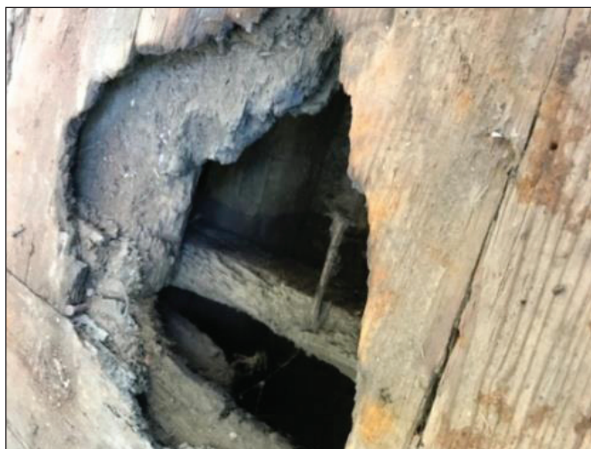
Photograph 24. This is the view of the layer under the sofa floor cover (mars mimarlık).
