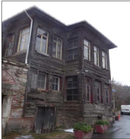
Photograph 21. This is the general view of the parsonage today.
