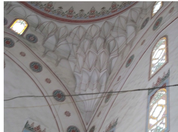
Fig. 8 Transition element, pendentive, of the main dome
