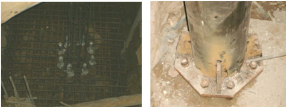
**Figure 13.** Circular columns anchorage
