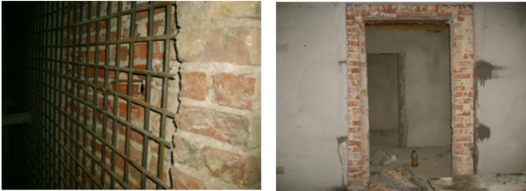
**Figure 11** Strengthening the walls
