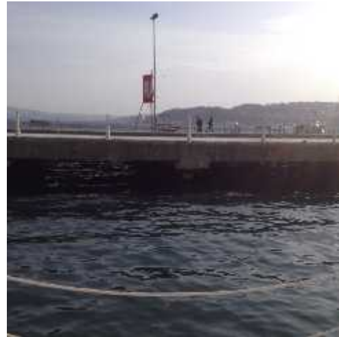
Picture 2. View of piled road in Sarıyer, 21/01/2014
