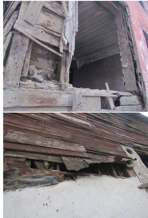
Figure 4.3: Former Architectural Feature of Sulukule; nogging structures with wooden frame
