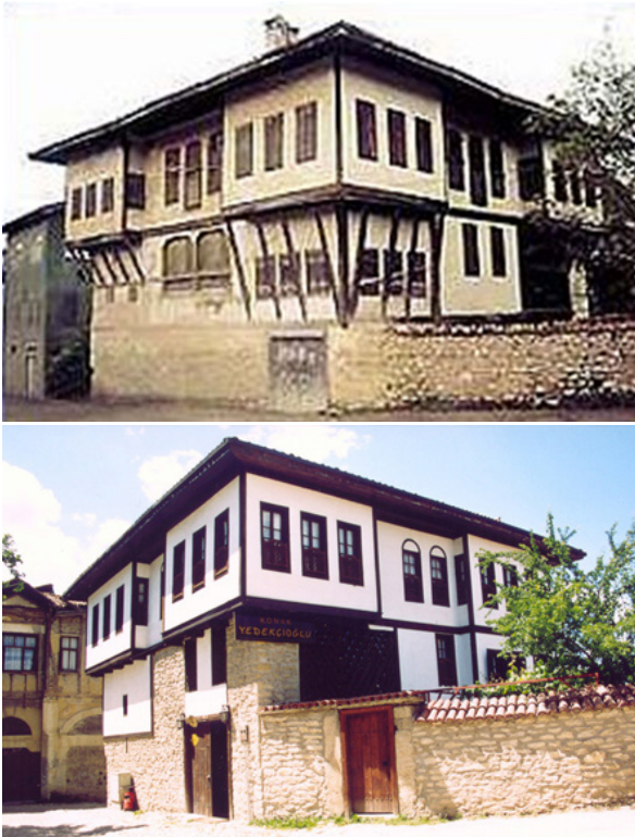
Figure 3.7 and 3.8: Appearance of a historical building in Safranbolu before and after the preservation attempts (www.forumcad.com) (www.karabukrehberi.net).
