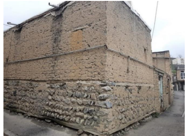
Figure 10. The materials of the envelope of a traditional building located in Tabriz.
