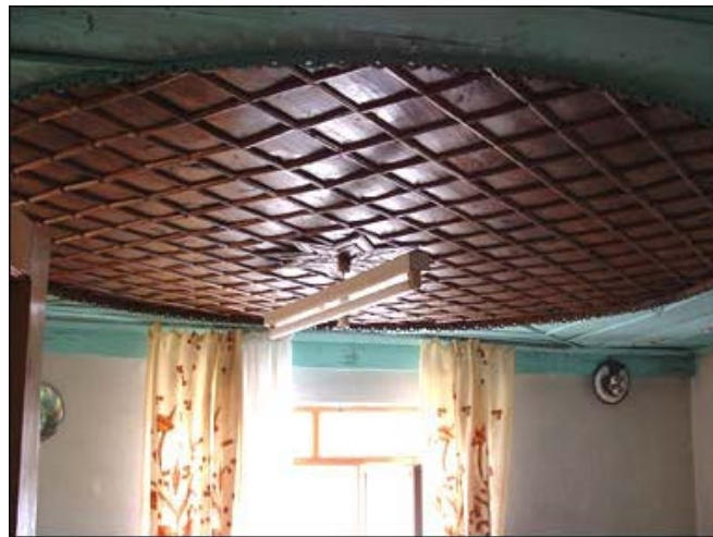
Figure 6. Durmus Yazici's buttoned house, southeast room ceiling view [9].
