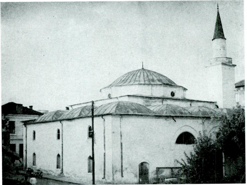
Fig. 9 — Jambol, Eski Cami. General view. Notice the enclosed “son cemaat yeri” and its walled-up arches
