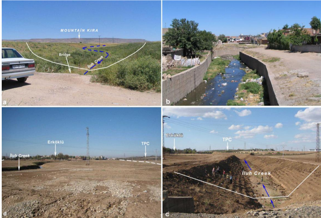
Photo 4. Morphological status of valley of Iluh Creek a) Valley of Iluh Creek east of Binaltlı. b) Canal of Iluh Creek in city center. c) Valley of Iluh Creek east of Erköklü before flood event on October 31-November 1, 2006. d) Earth-lined canal of Iluh Creek constructed east of Erköklü before the flood event.
