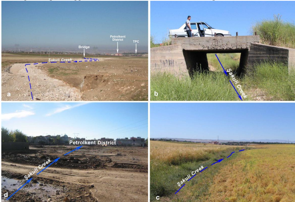
Photo 6. Şakuli creek, affecting the south part of Batman city. a) Stream bed of Şakuli creek on the alluvial fan to the south of west Mount Raman.
