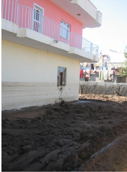
Photo 3. Aggregations of mud up to 1 m high observed in the gardens of some houses as a result of the flood and torrent event in Batman on October 31-November 1, 2006.
