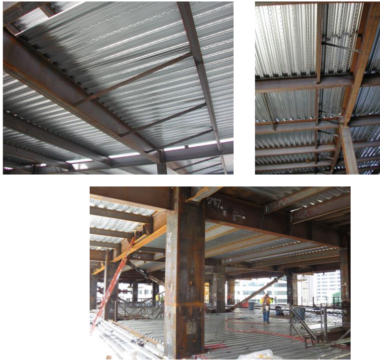
Figure 8 Beam Bracing Samples
