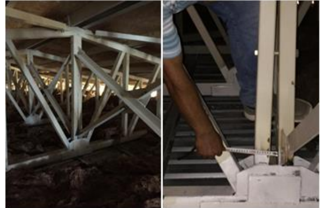
Figure 2. Roof trusses manufactured in two parts
