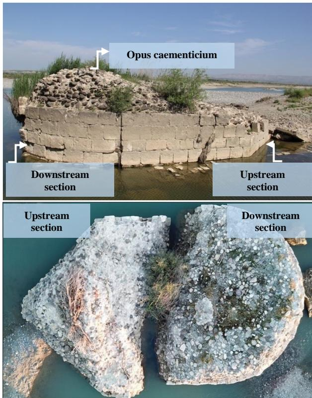
Figure 4. Different views from the piers/foundations
