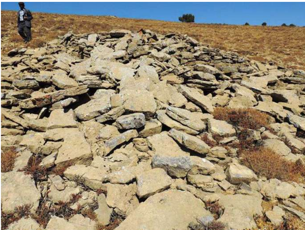
Fig. 40 One of the destroyed construction.
