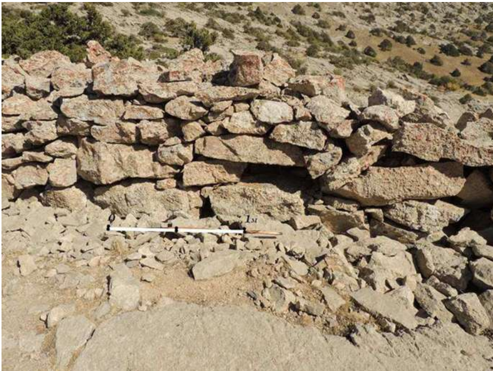
Fig. 20 Base of preserved part of shahristan wall.
