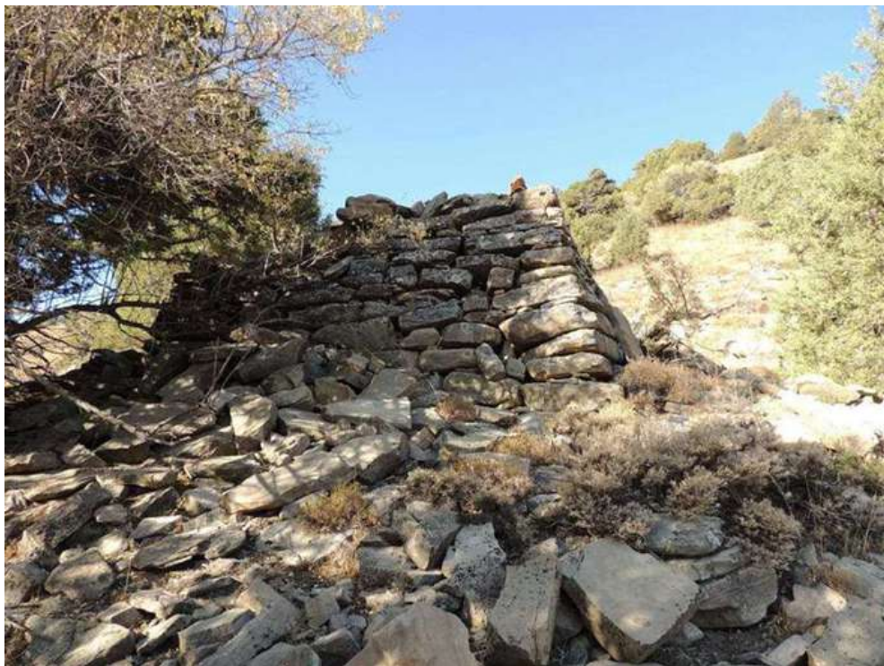
Fig. 34 Construction no 13 eastern side.
