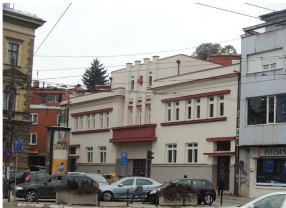
Figure 9. The Red Cross building, Kranjčevića ulica, Sarajevo; After the full reconstruction (2013-2017).
