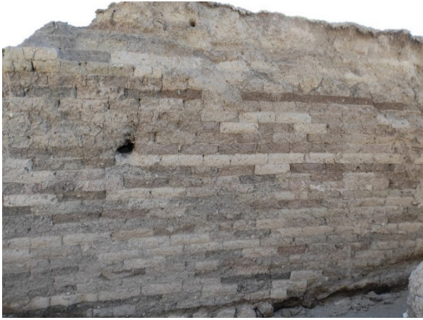
Fig. 16. Upper Anzaf, a current view of a section of the Northern Corridor wall (Courtesy of Vedat Timur).
