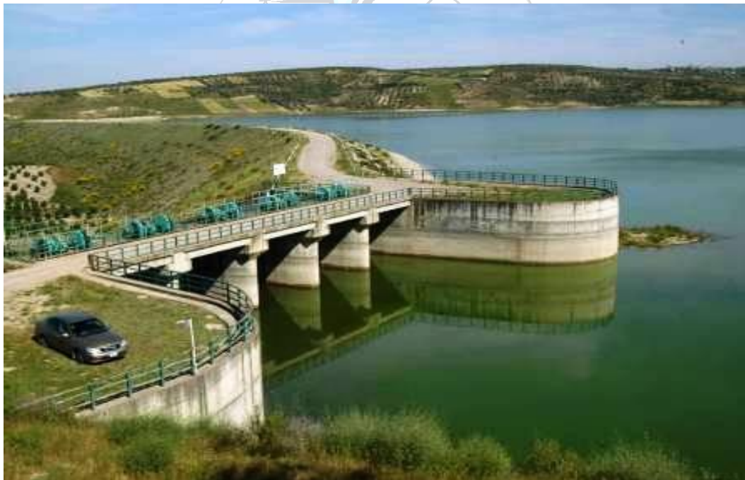
Figure 2. General view of Yarseli dam
