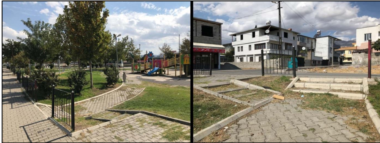
Figure 3. Ramps and stairs
